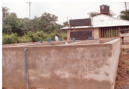
New Recirculatory System for fingerlings Development
